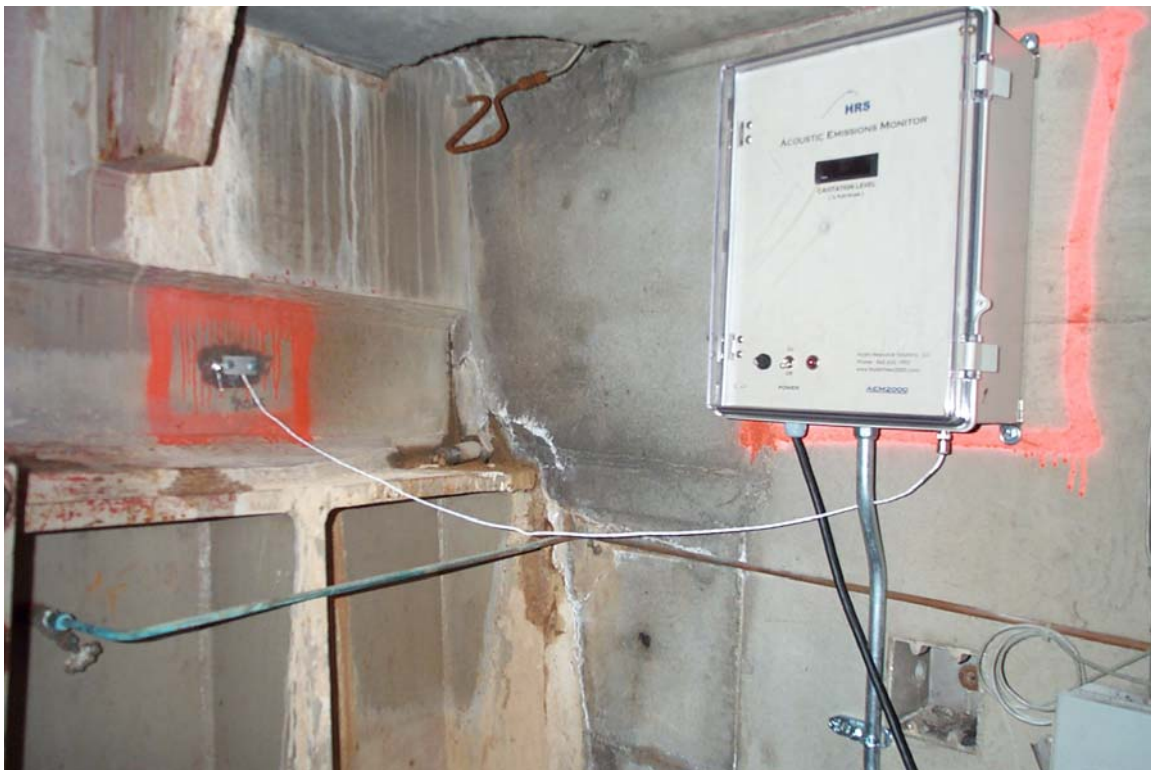
Figure 1: AEM2000 Installation on G-24
